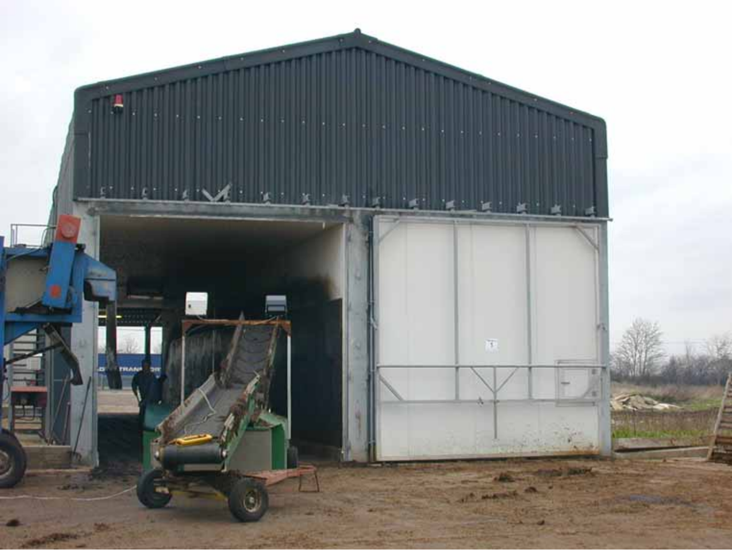
Figure 1: Gicom batch composting tunnels – concrete and steel construction - with filling equipment
