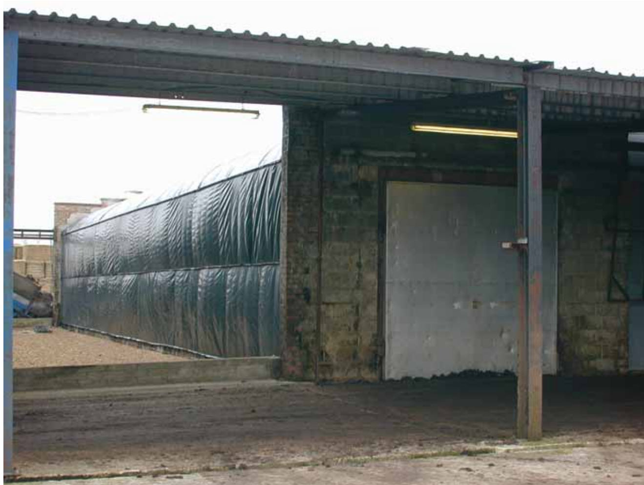
Figure 2: Poly-tunnel batch composting tunnel – concrete internal walls and insulated poly-tunnel cover
